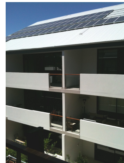
Square One - 14 Money Street, Perth Master Builders Award 2010 for Energy Efficiency and Sustainability
